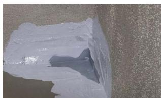
Alternatively, you can reinforce inner corners using a tailored piece of the KÖSTER Superfleece, measuring approx. 20 cm in length. Fold this fabric strip in the middle and make a centered cut halfway through. This prepared
