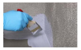
mend using the pre-fabricated accessories in critical areas. These include the corners, junctions, floor drain and wall penetrations.
