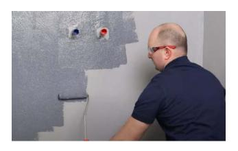
KÖSTER BD 50 is applied to the entire on the wall and floor surface using a roller or a brush. To minimize disruption and ensure a flawless application, it is recommended to begin by waterproofing all the walls and conclude with the floor areas.
