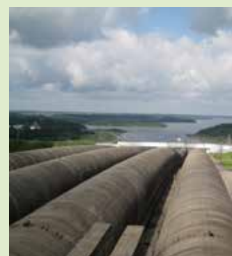
Water power plant, Lithuania
